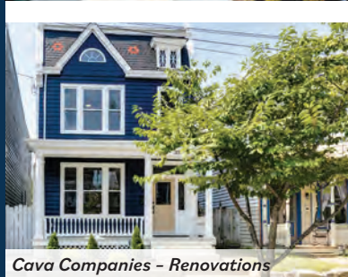
Cava Companies - Renovations
